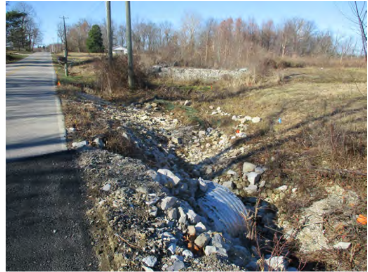
12.) Culvert crossing from protected wetland
