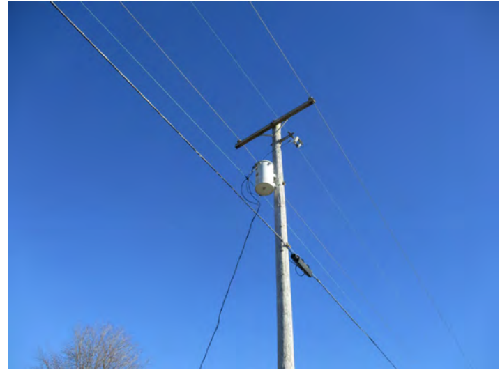
4.) Single-phase pole transformer (S-PPT) near SE p.c.
