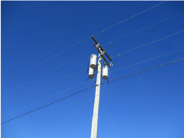
7.) Three-phase pole transformer east of pump station
