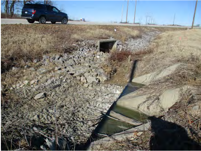
41.) Pond overflow and culvert crossing underneath Highway 57
